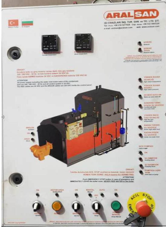
**Conventional control panel is used between 50 kg/h to 800 kg/h**
